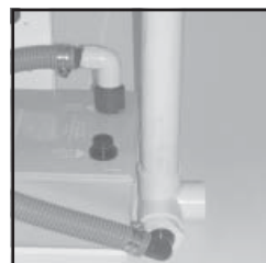
Drain tube installed
