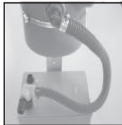
Overflow Tube Installed
