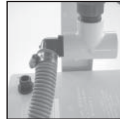
Expansion Tee Installed
